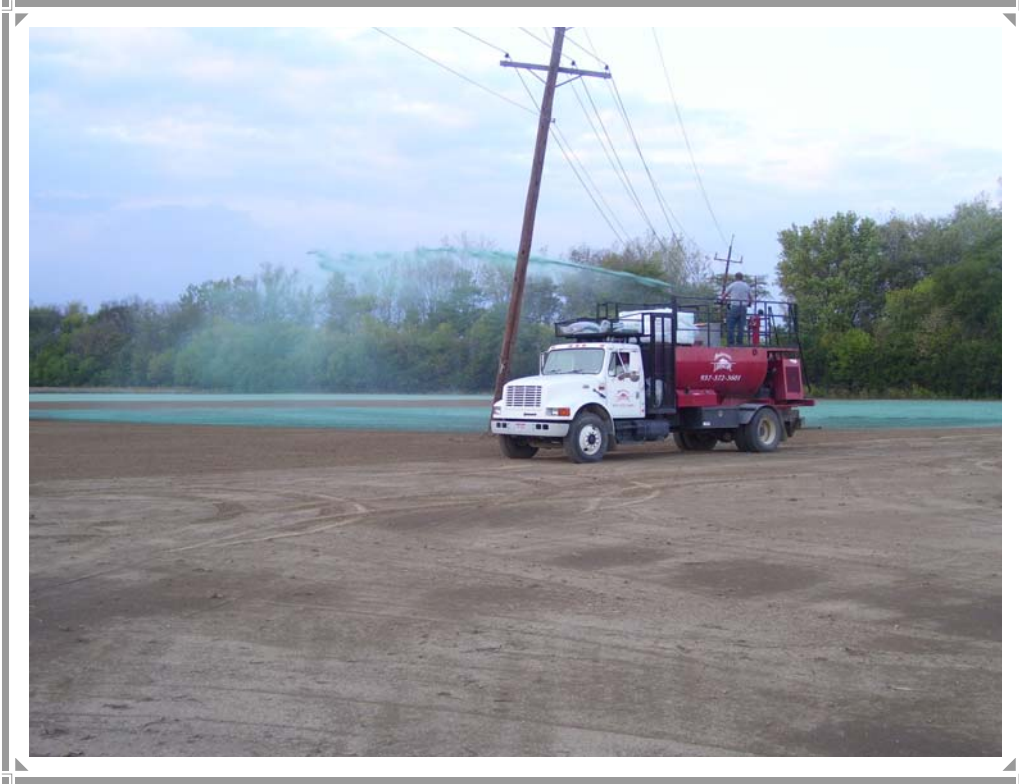
The surface application process (hydro-seeding) is ongoing and will be completed Oct. 5, 2007.
