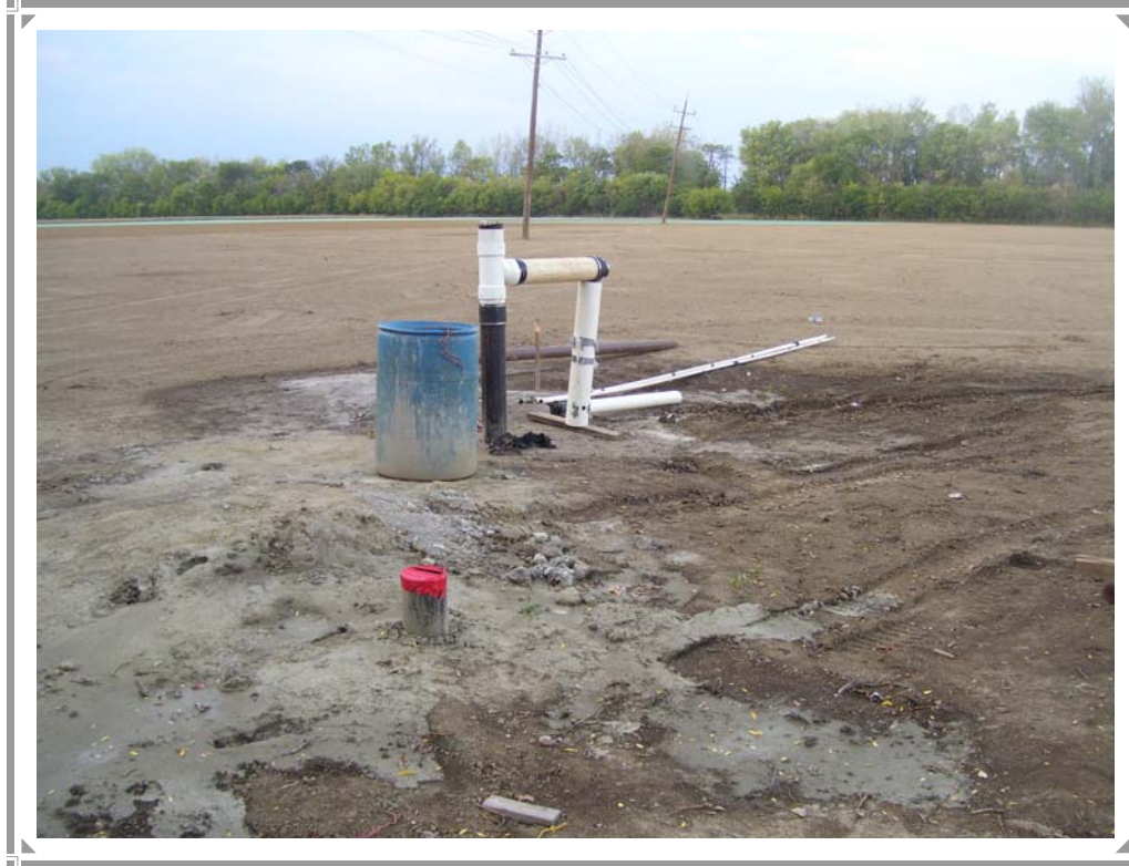
The irrigation well is one of the most important parts of the project. It will provide water to the facility for years to come. Upon completion the well should provide over 100 gallons of water per minute to the fields. The facility will be watered using a walking reel.
